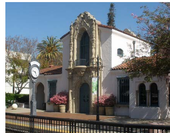
Claremont Metrolink Station (Category #6) Claremont, CA
